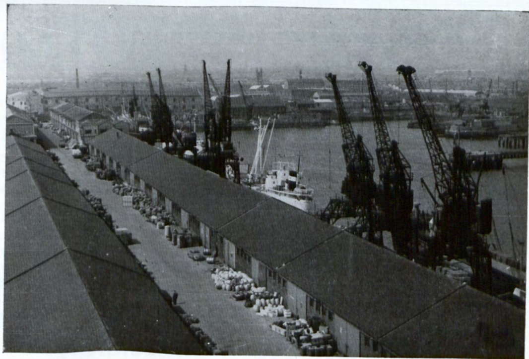
North Wall Extension
